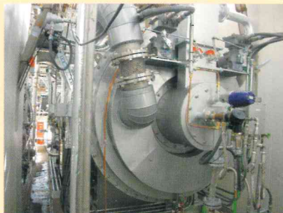
蒸発濃縮式廃液減容化装置 Evaporation type waste fluid concentrate equipment
