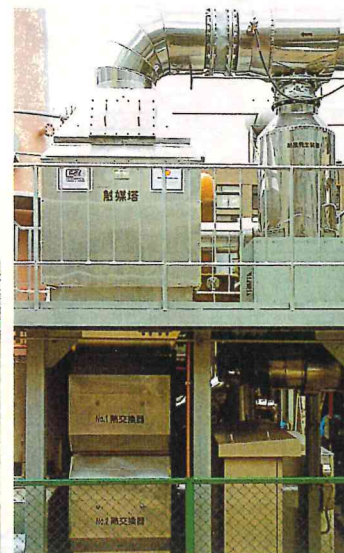
触媒塔 Catalytic reactor
