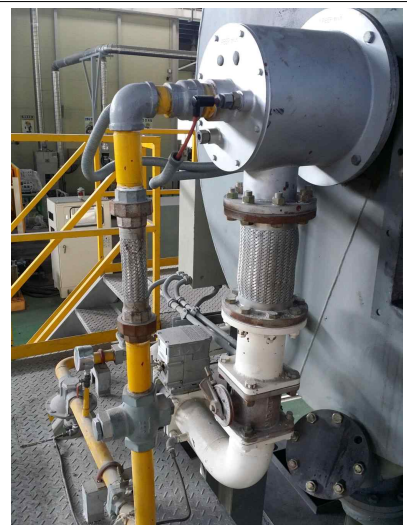
2-22. Rist-Gas burner 80만kcal/hr
